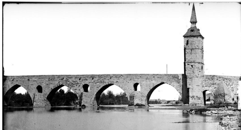
Figure 2. Bridge over the Duero river in Zamora, photograph acquired by J. Laurent, in 1870. Photograph of the southern half (arcs 7–3).
