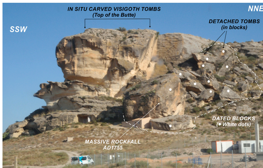
Fig. 6. Photograph of the rockfall affecting calcarenitic rocks in the “Tolmo de Minateda”, displaying the position of collapsed largest blocks and carved visigothic tombs. After Pérez-López et al. (2019).
