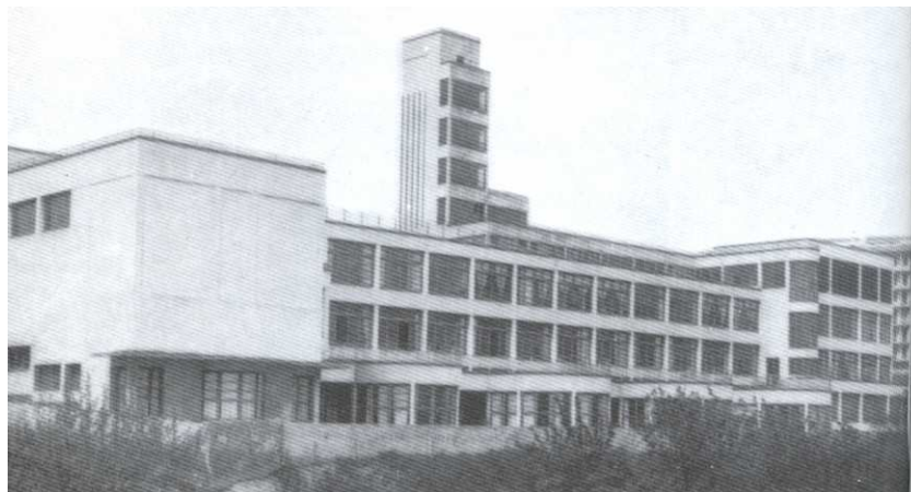
9. Pedro Ispizúa, architect, 1932-1933. Briñas school, Bilbao.
