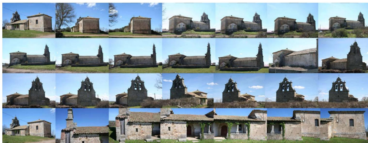
Figure 3. Images following a “ring” shot strategy around the parish church of Ceadea.
