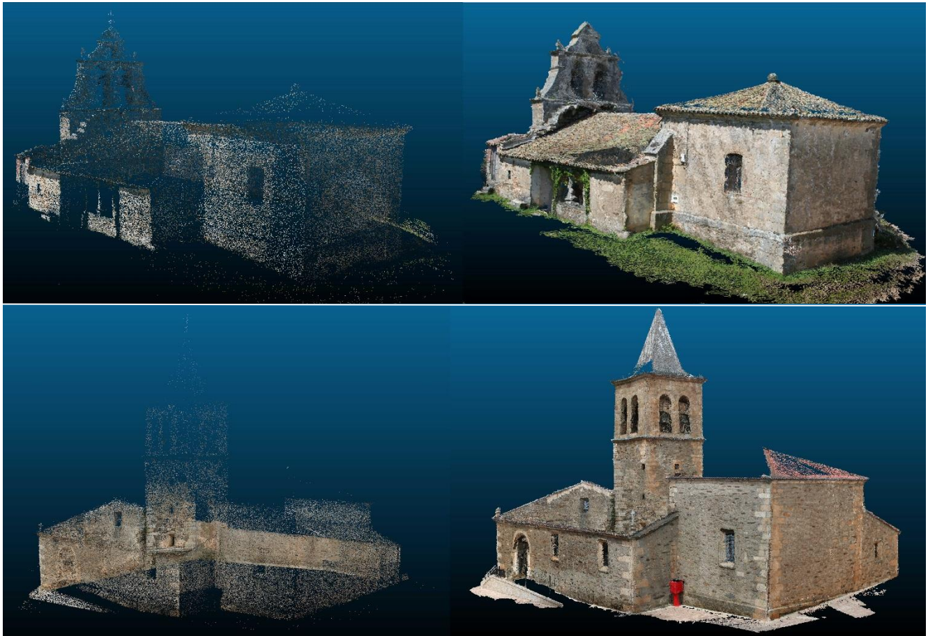
Figure 5. Scattered point cloud from the matching process ( left ) and dense point cloud from the SGM or PMVS strategy ( right ). The parish church in Ceadea ( top ) and the parish church in Trabazos ( bottom ).
