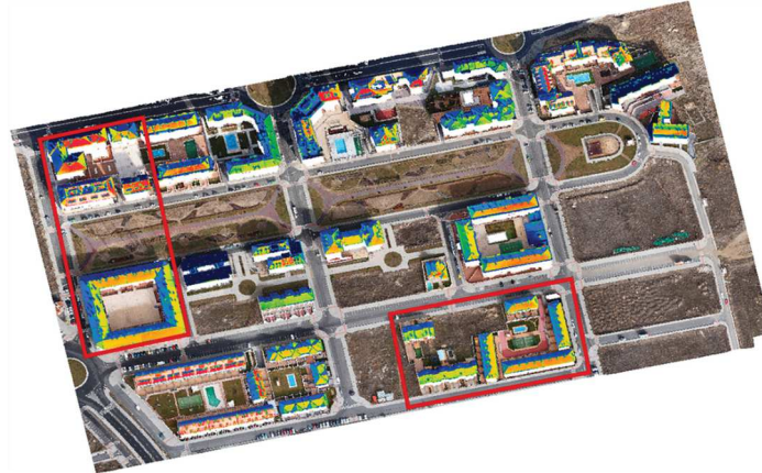
Figure 7. Hybrid 3D point cloud generated from images captured with the RGB camera integrating thermographic texture mapped over the roofs. Areas shown in detail in consecutive figures are remarked in red.
