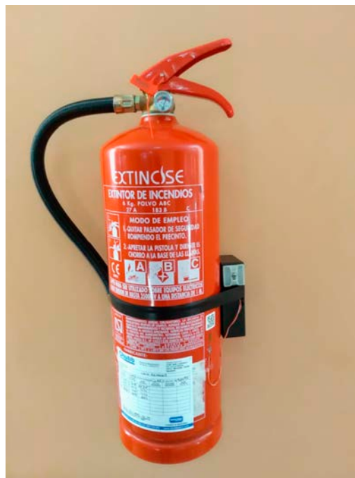
Figure 10. A SmartFire prototype situated in a fire extinguisher in the building of the case study.
