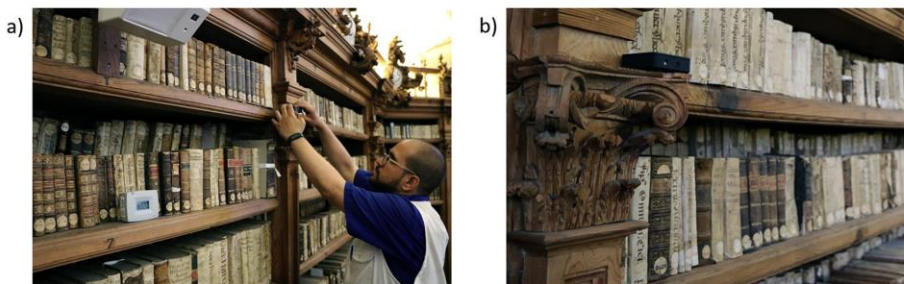
Fig. 14. Nodes installation in the Library.
