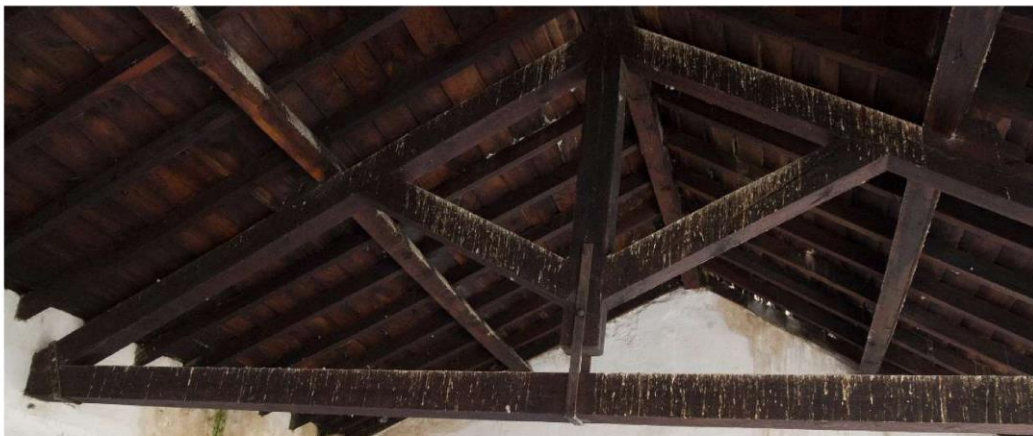
Figure 6. Gallery; detail of an open-node truss.
