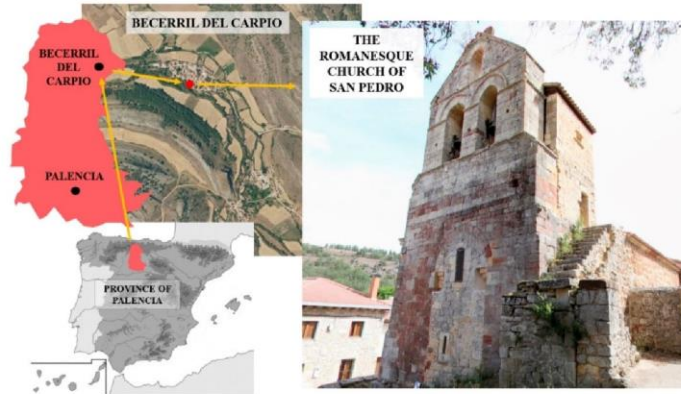
Figure 1. Location of the Romanesque church of San Pedro (Becerril del Carpio, Spain).
