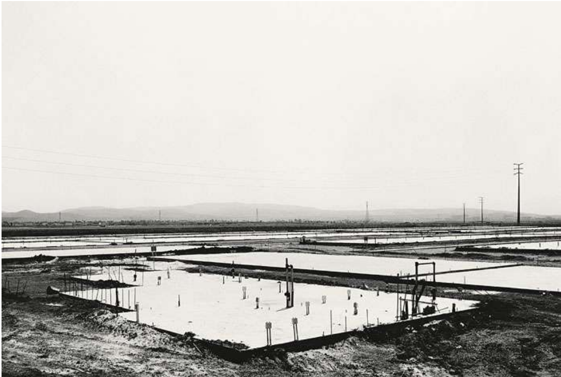
Fig.7. Baltz, Lewis. Foundation Construction, Many Warehouses, 2891 Kelvin, Irvine, 1974 . De la serie The New Industrial Parks near Irvine, California . ©The Lewis Baltz Trust.
