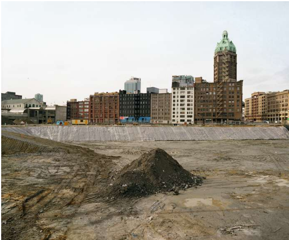
Fig. 14. Arden, Roy. Construction Site and Suntower , Vancouver BC, 1992. © Roy Arden.
