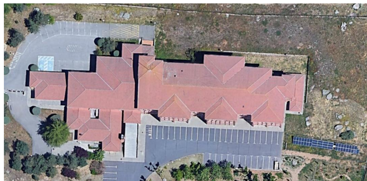
Figure 1. View of the University School of Education and Tourism together with the 10 kW photovoltaic installation visible on the right.
