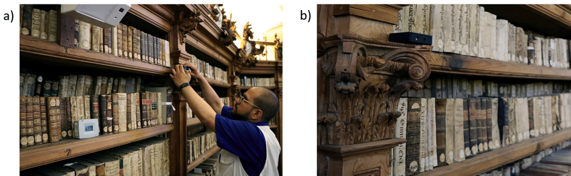
Fig. 14. Nodes installation in the Library.
