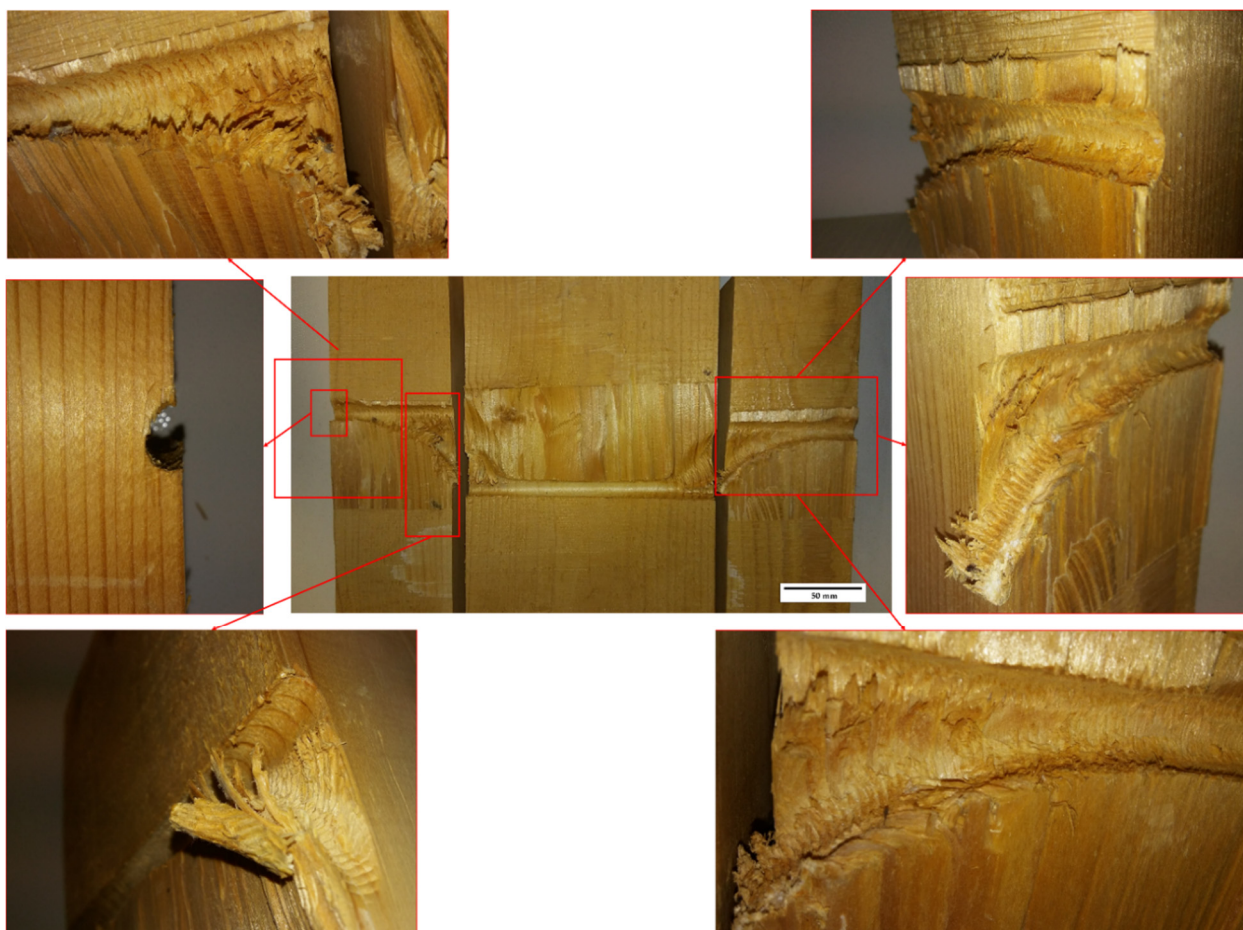
Figure 15. Condition of the timber after the test with dowel without washer nut fixing ends. In the external areas, the wood has crushed due to the dragging of the threaded dowel and when the displacement grows, the threaded dowel is embedded in the timber, causing clawing or gripping and contributing to the rope effect.
