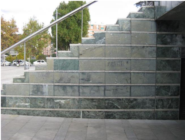
10 11 12 13 14 15 16 17 18 19 20 21 22 23 24 25 26 27 28 29 Fig. 1. Unattractive visual appearance of serpentinite slabs with different chromatic characteristics placed 30 on the exterior the Granada Exhibition and Convention Centre
