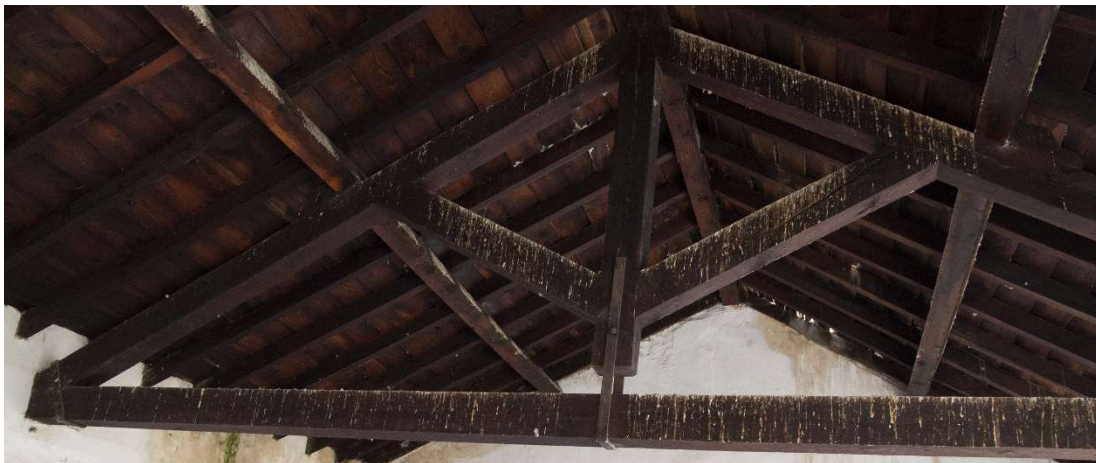
Figure 6. Gallery; detail of an open-node truss.
