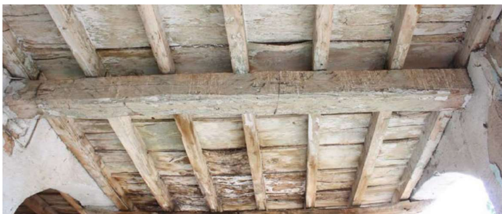
Figure 7. Internal cloister; detail of a wooden floor with a double row of beams and overlapping joists.
