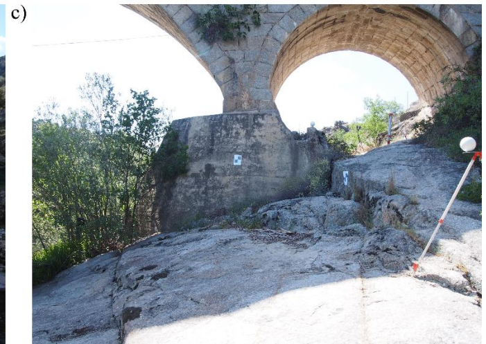
Figure 1: The Arco Bridge: a) downstream elevation before and after restoration works; b) upstream elevation and; c) reinforced concrete layer added to the pier between vaults.
