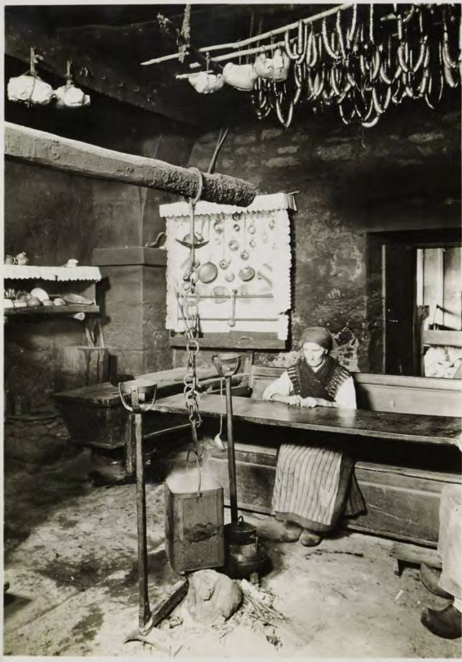
Anderson 1887 Kitchens Corgo Lugo
