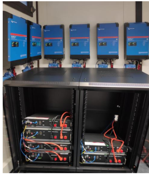
Figure 3. A real BESS from GECAD/ISEP was used for implementing the proposed methodology.
