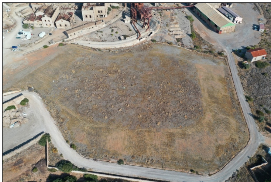
Figure 4. Hazardous-waste landfill located at the LTCP.
