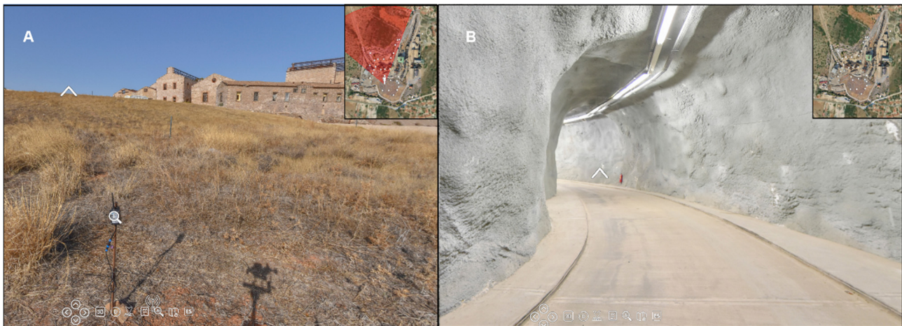
Figure 20. Captured views from the virtual tour of the LTCP infrastructure. (A) External deposit area showing the deployment of IoT sensor nodes. (B) Section of the underground gallery network.
