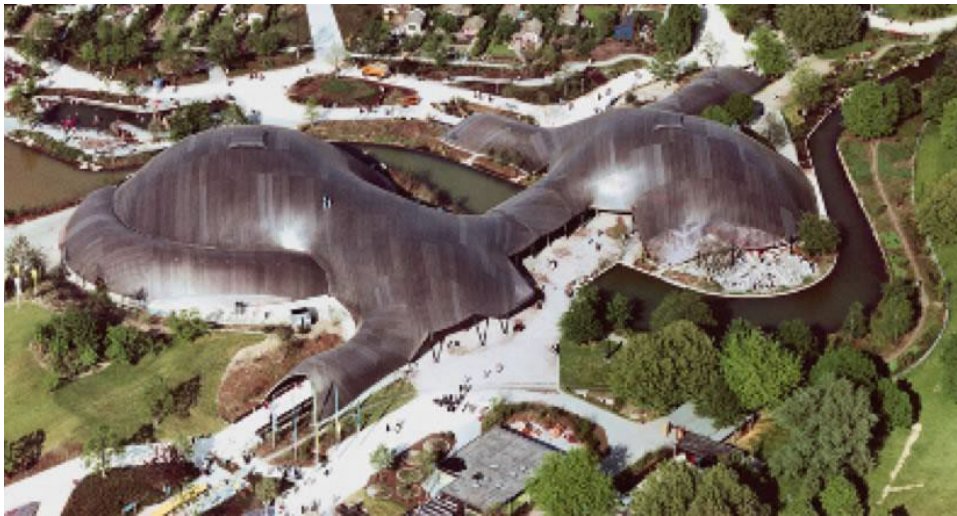
Fig. 221. Centro Multifuncional de Mannheim. Fuente: https://www.designboom.com/architecture/frei-otto-a-life-of-research-construction-and-inspiration-detail-book-report-06-02-2015/.jpeg
