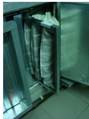
Figure 49 - Filter class F8
