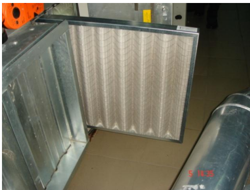
Figure 48 - Pre-filters class G4
