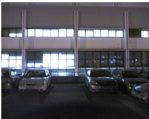
Figure 39 - Picture of Building D
