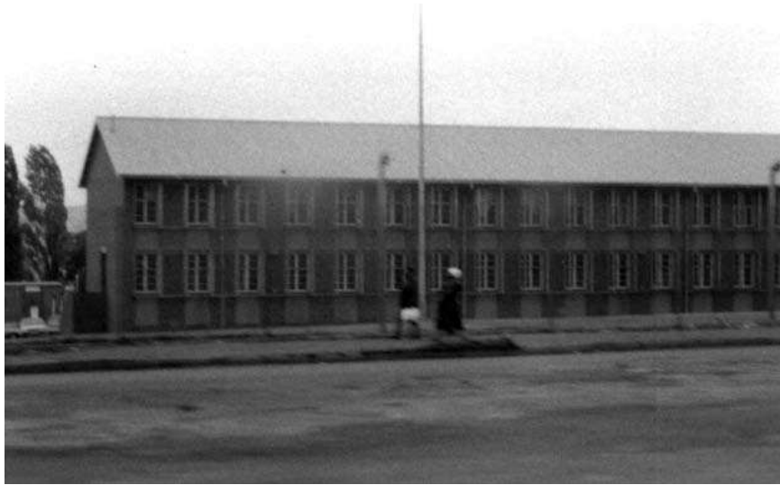
Hostel Compound, Soweto, South Africa, 1989
