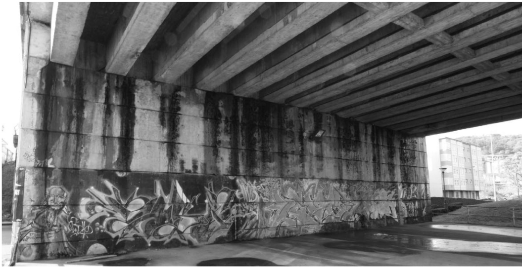
Figure 13.2 Pier of the Ribeiriño bridge.
