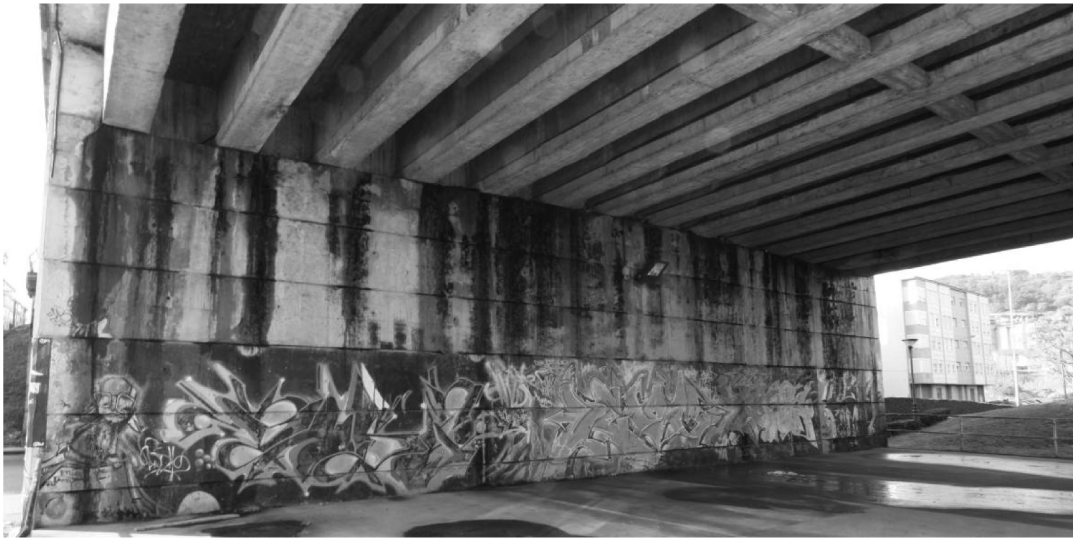
Figure 13.2 Pier of the Ribeiriño bridge.
