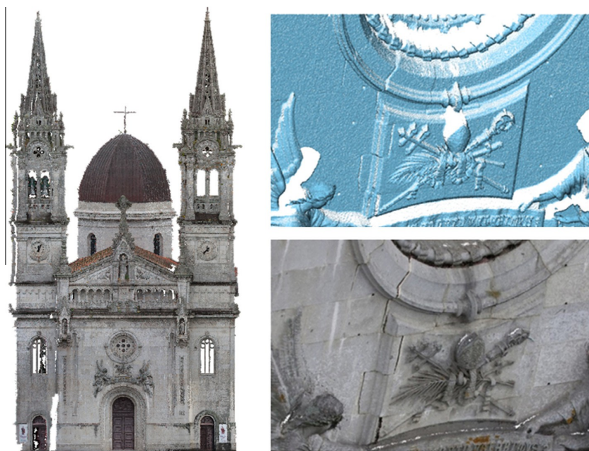
Fig. 7. Front elevation of the point cloud obtained through SfM technique and PW software (left). Detailed comparison between the laser scanner point cloud and the one obtained in PW software (right).
