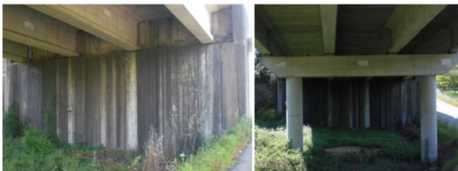
Figure 8. Images of a wall of the abutment studied.
