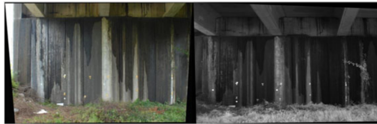
Figure 10. Camera images corrected for perspective. On the left is an RGB image and on the right a band 0 image (778 nm) from the MCA6.
