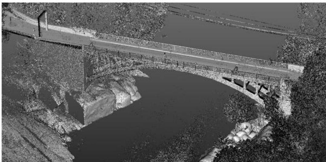
Fig. 9. 3D representation of the bridge resulting of the point cloud optimization.
