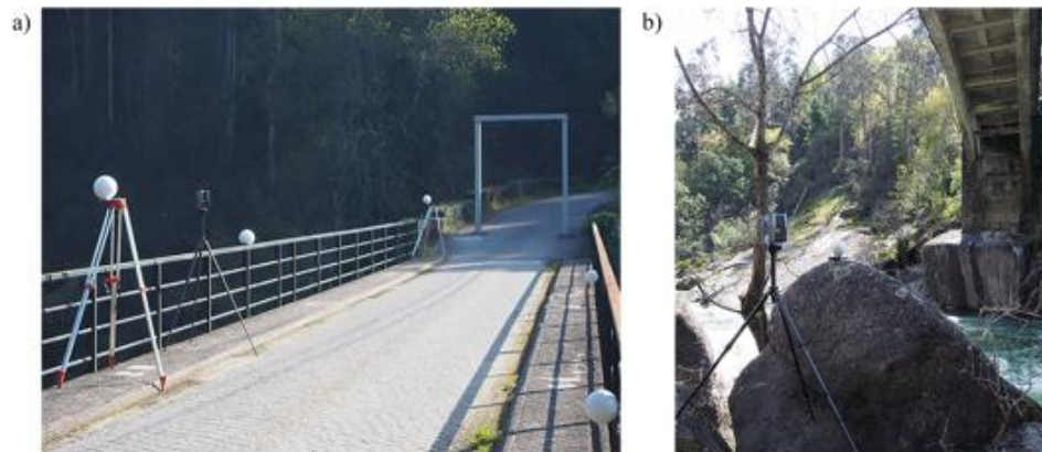
Fig. 8. TLS and registration spheres used during the data acquisition: a) during the recording of the deck; and b) TLS surveying at the lower part of the bridge.
