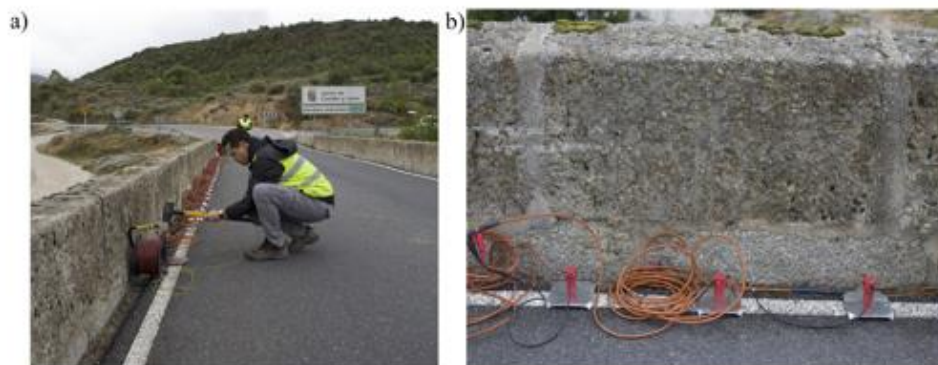
Fig. 6. MASW test carried out on the bridge: a) instrumental hammer and b) geophones with a natural frequency of 4.5 Hz.
