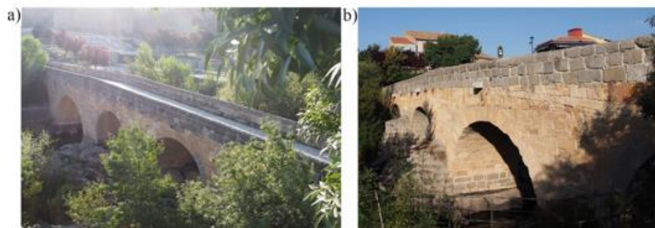
Fig. 1. General view of the bridge: a) upstream and; b) downstream.
