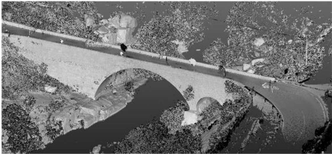
Fig. 11. 3D representation of the optimized point cloud of the bridge.
