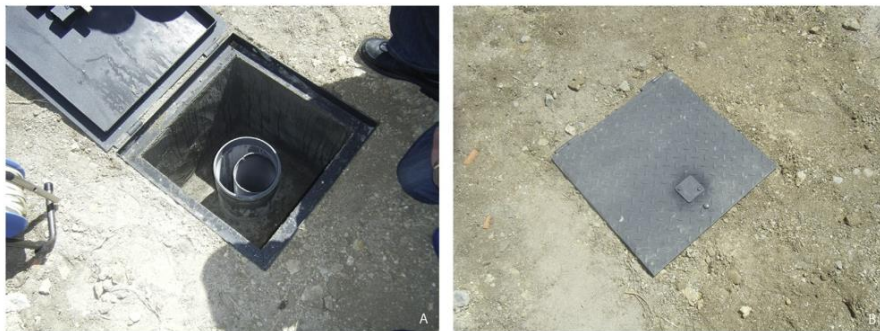
Fig. 5. Stage 3. (a) Placing of the manhole. (b) Closing of the hole.
