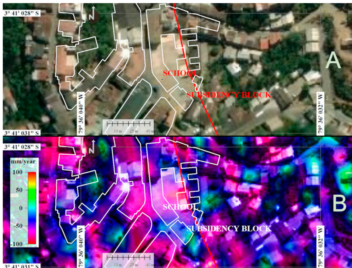
Figure 9. (A) Location of Fe y Alegría-La Inmaculada School in the study area before the collapse of the block of school classrooms. (B) Block collapse of school classrooms on October 25 of a day before the collapse that began on October 16, 2016, and completely collapsed in December 2016. The faint blue color indicates that before October 25, 2016 the sinking of the area was in process. Gallery is in red color and blocks houses are in white color.
